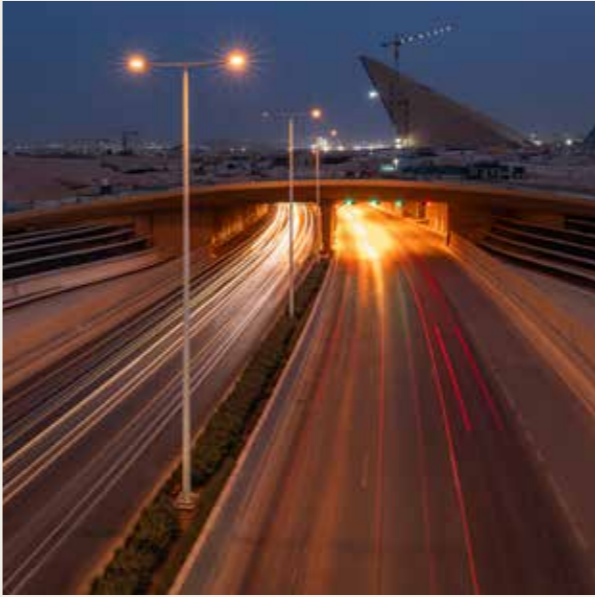
2.5 km Tunnel Diverting Traffic Under the Park
