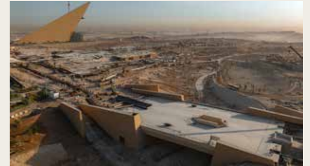
The Loop Bridge | Current Progress
