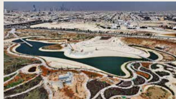
Art Park | Current Progress
