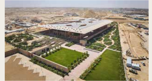
Visitors Pavilion | Current Progress
