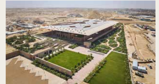
Visitor Pavilion | Current Progress 100% complete
