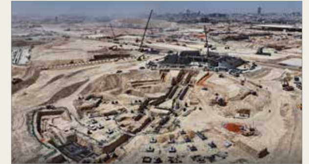
Central Forest: Amphitheater | Current Progress
