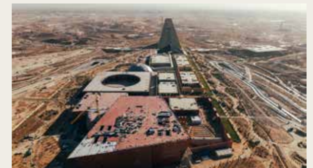
Royal Arts Complex | Current Progress 87% complete
