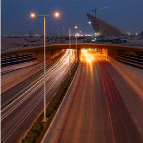
2.5 km Tunnel Diverting Traffic Under the Park
